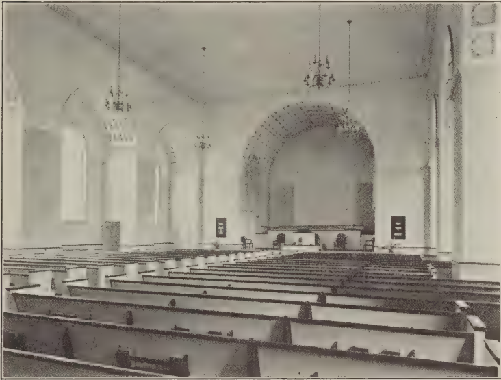
INTERIOR OF MAIN AUDITORIUM OF FIRST M. E. CHURCH, SOUTH, CHARLOTTESVILLE, VIRGINIA
